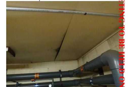
Figure 1.30, Mechanical room ceiling damage
