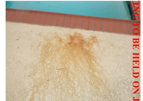
Figure 1.18, Pool deck corrosion
