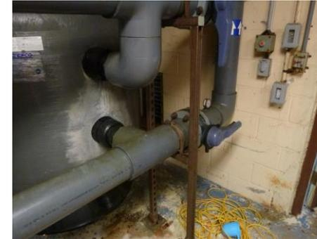
Figure 1.34, Piping support corrosion | area of filter leak
