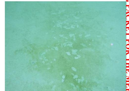
Figure 1.4, Plaster surface etching/delamination
