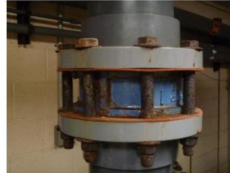
Figure 1.33, Piping bolt corrosion
