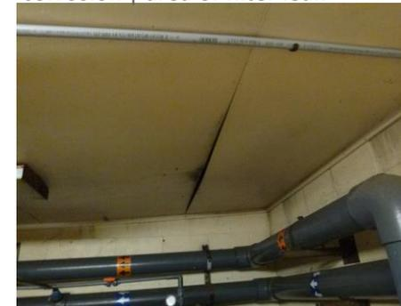
Figure 1.42 Mechanical room ceiling damage
