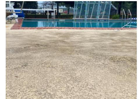
Figure 1.12, Uneven/shifting concrete deck and pool
