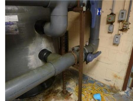
Figure 1.40, Piping support corrosion | area of filter leak
