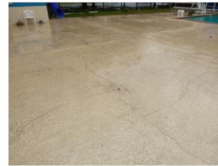
Figure 1.19, Pool deck cracking
