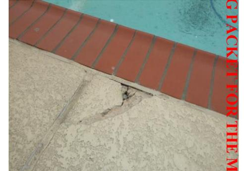
Figure 1.16, Pool deck delamination
