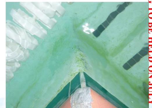
Figure 1.6, Cracking, delamination on corner
