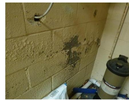
Figure 1.38, Mechanical room wall deterioration
