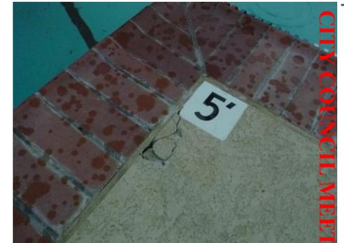
Figure 1.14, Pool deck delamination
