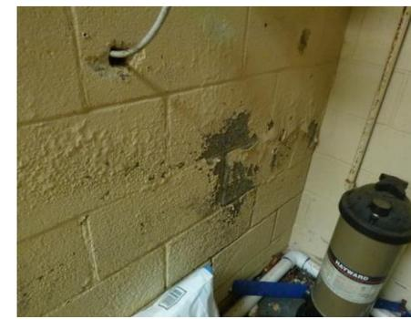
Figure 1.32, Mechanical room wall deterioration
