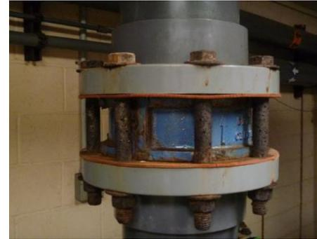
Figure 1.39, Piping bolt corrosion
