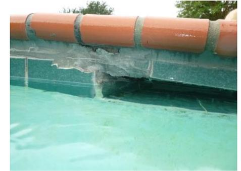
Figure 1.10, Cracked, shifting skimmer basket
