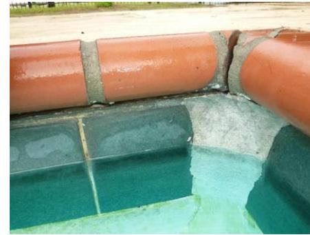
Figure 1.7, Coping stone loose and cracking
