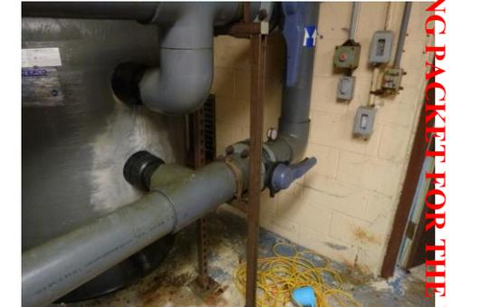
Figure 1.28, Piping support corrosion | area of filter leak
